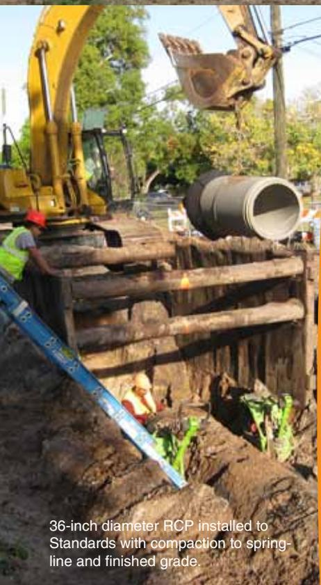
36-inch diameter RCP installed to Standards with compaction to spring-line and finished grade.
