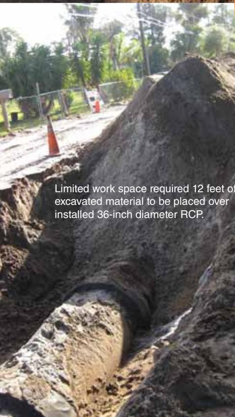
Limited work space required 12 feet of excavated material to be placed over installed 36-inch diameter RCP.
