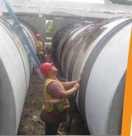
A Pipe Tugger assists with homing 96-inch diameter O-ring gasketed joints.
