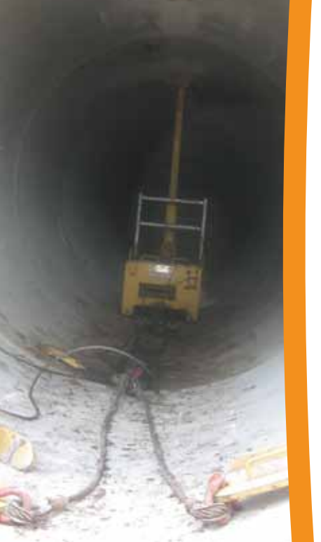
Pipeline Utilities developed a handheld device to compact haunches of large diameter and elliptical pipes.
